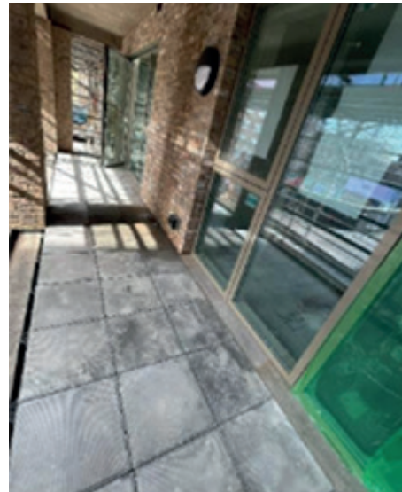
Aytoun Road Show Flat Progress of Works Balcony
