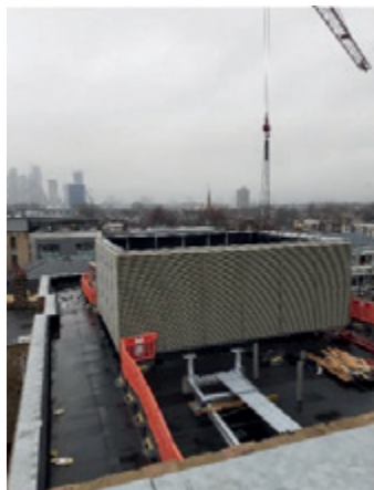
Aytoun Road installation of Air Source Heat Pump Enclosure
